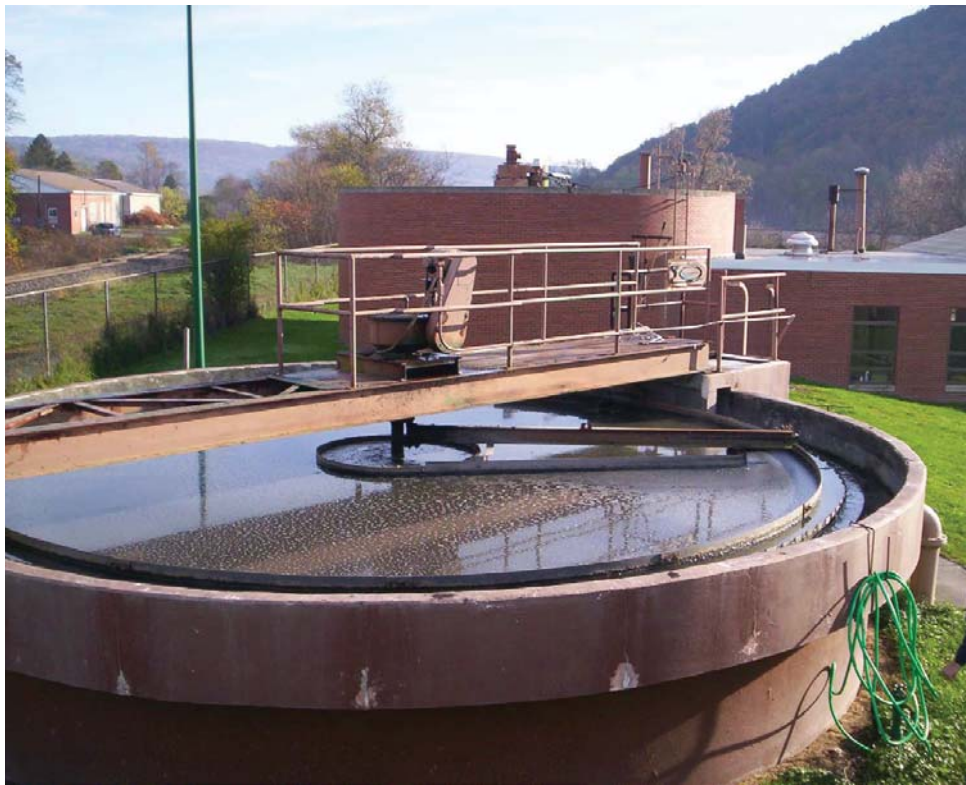
CLARIFIER PRE-CONSTRUCTION AT ADDISON, WORN GEARBOX, CRACKED WALLS AND A WORN ARM THAT WOULD OFTEN STICK
